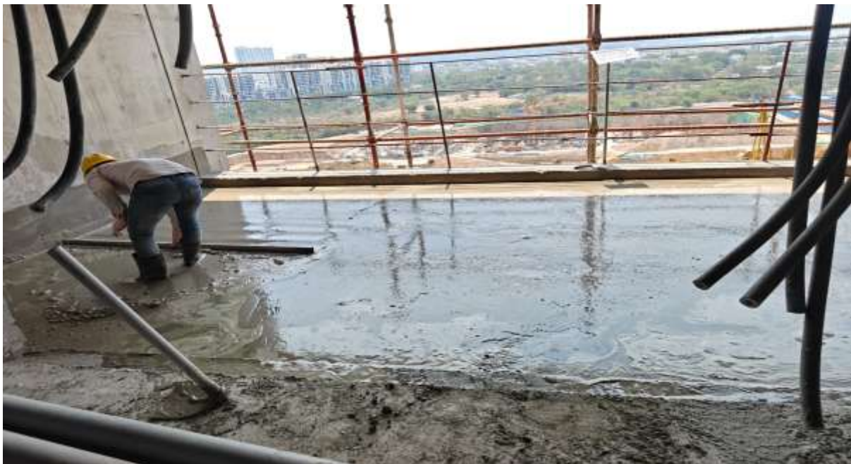
(Figure 7.2: Level Finishing Activity )
