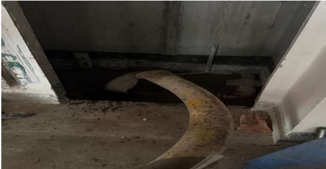
(Figure 7.1: Foam Concrete Pumping Activity )
