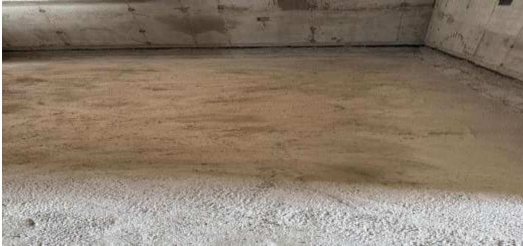
(Figure 11.1: Finished Foam Concrete Surface )
